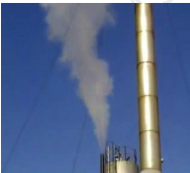
Conventional Traps : Huge flash steam cloud
